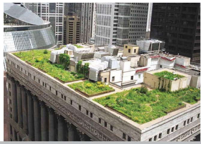
Chicago's City Hall was retrofitted with a green roof in 2000.
